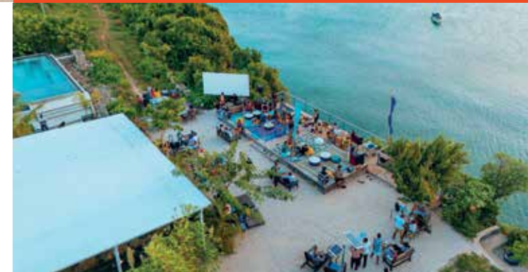
Fumba Town got a first public pool recently and long awaited street paving is progressing. The seaside suburb of Zanzibar City is using a modern variation of cobblestones. Green builders prefer them to tarmac roads because they allow rainwater to sink into the soil. The first public pool in Fumba with spectacular seaside views was opened near the Kwetu Kwenu Chill restaurant (photo).
