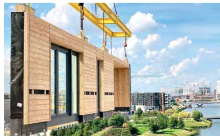
Critical moments: entire walls with windows are lifted during construction
