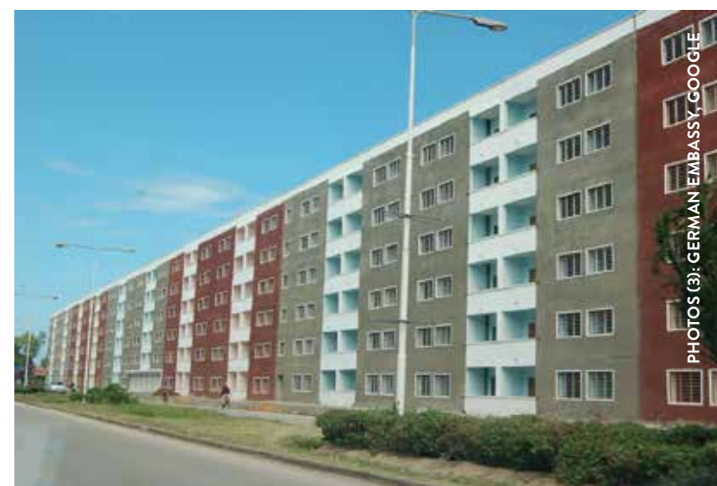
A gift from East Germany in the 1970s: The Michenzani flats in Zanzibar, meanwhile flanked by a new shopping mall opened in 2021. The area around the "German flats" is earmarked for major modernisation
