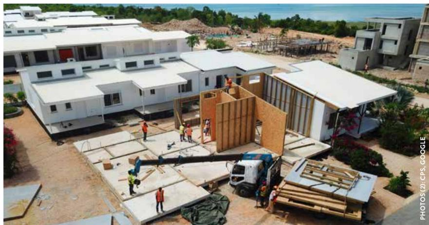
Fast forward: It takes only a week to a month to assemble a prefab timber frame house, like this family home in Fumba. Another advantage is that unlike cement, wood waste can be composted
